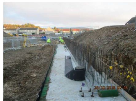
4 Retaining wall base
