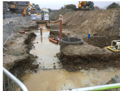
2 Drainage works to the site of the new school building
