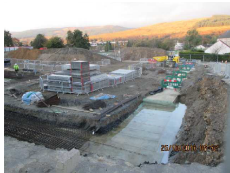
7 Sports Hall footprint following drainage works
