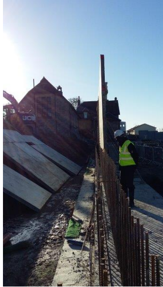
5 Reinforcement to the retaining wall
