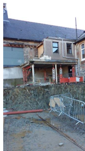
8 Additional structural support added to the rear of 1881 building
